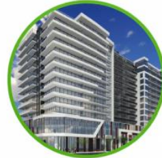
212 King William Street Approved | 14-storey building with commercial uses and 266 dwelling units.
