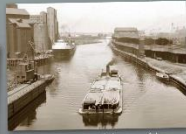
Grain elevators were signal elements of the Buffalo skyline. They received Midwestern grain from lake freighters, stored it, and then shipped it to canal boats and rail cars for distribution to New York City and the world beyond.
