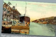
Rail cars emptied their loads of bituminous coal onto upper levels of trestles that angled into Buffalo harbor. Grey-rod chimneys loaded canal boats that hauled east across New York and Lake vessels that carried fuel to Midwestern industries and homes.
