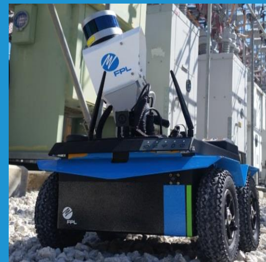
Autonomous Substation Robot
