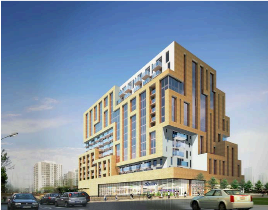
299 Campbell Street – Under Construction Toronto ON
